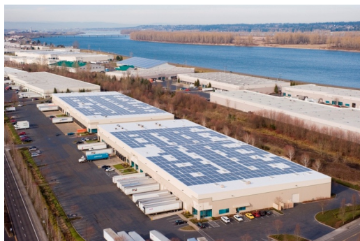
ProLogis / Portland Electric , Portland, Oregon, USA, 3,5 MWp
